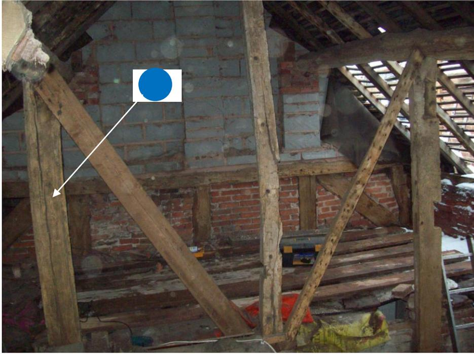
Figure 4g: View of partition frame 5b to show sampled timber (colour coded by felling date/range). Parts of the remaining portions of truss 6 may be seen just beyond it
