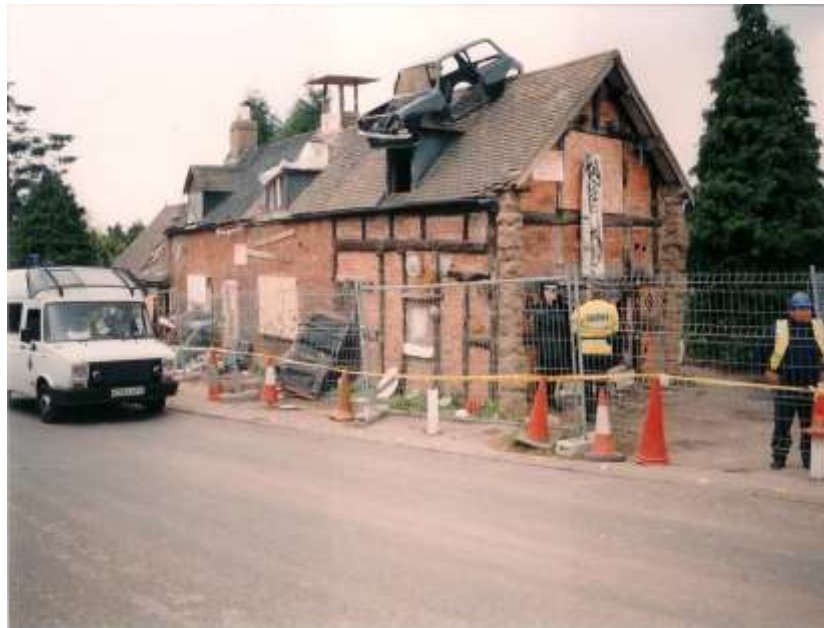
The scene on Tuesday 14th April 1998. The police had secured the site and contractors were about to arrange for ‘Boundary Cottage’ to be demolished.
