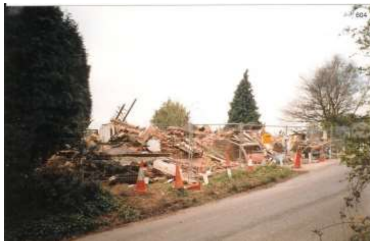
Further view of the demolished cottage.
