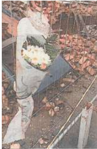
Flower tributes on the fencing outside the demolished 'Boundary Cottage', on Wednesday 15th April 1998.
