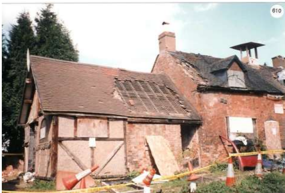
Another view of the cottage, shortly after the eco-warriors had vacated the building.
