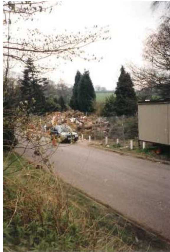
'Boundary Cottage', following its demolition on the Wednesday.
