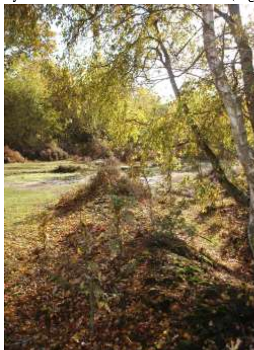
Fig. 7 – Looking in the opposite direction towards Pool Hollies. Much of the earthbank is colonised by Birch and heather.
