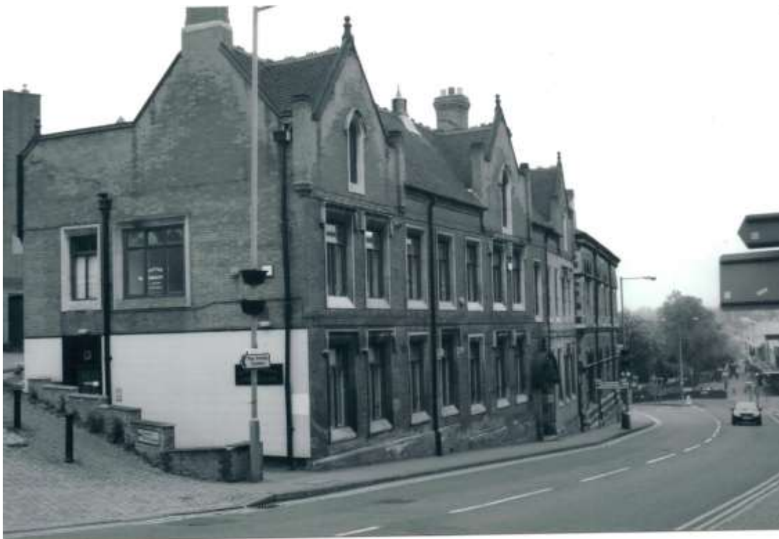
The former workhouse building in Mill Street
