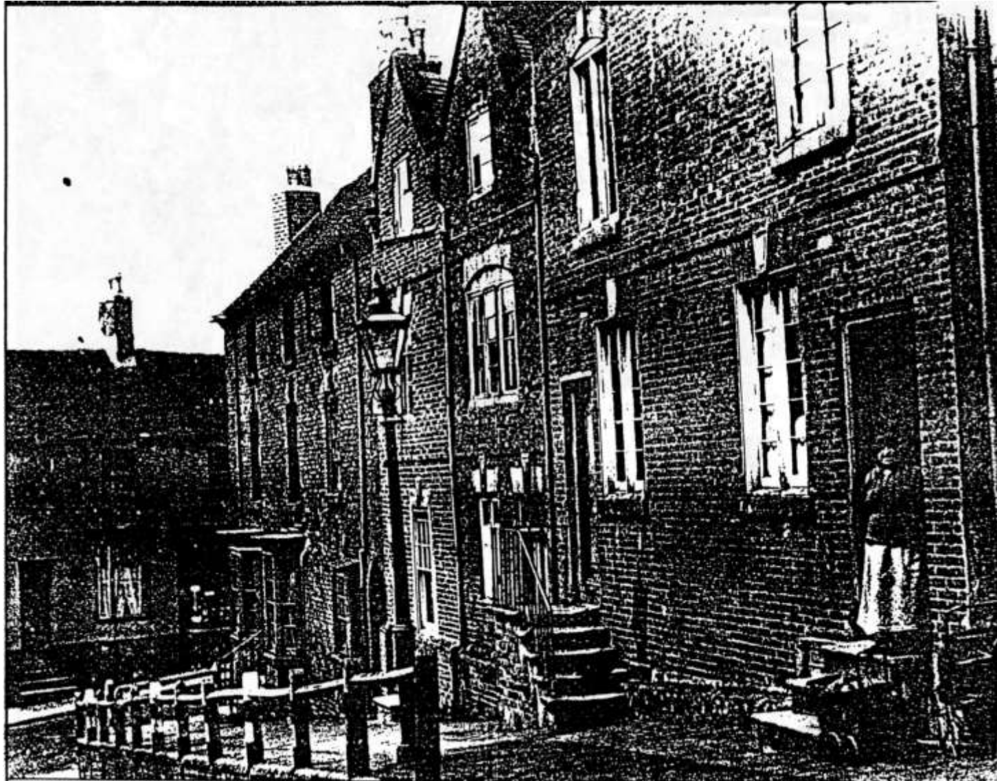
Gas Lamp on Church Hill Sutton Coldfield Erected 1871
