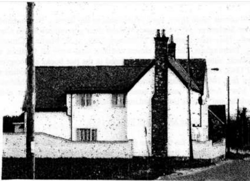
Ash Cottage — west elevation
