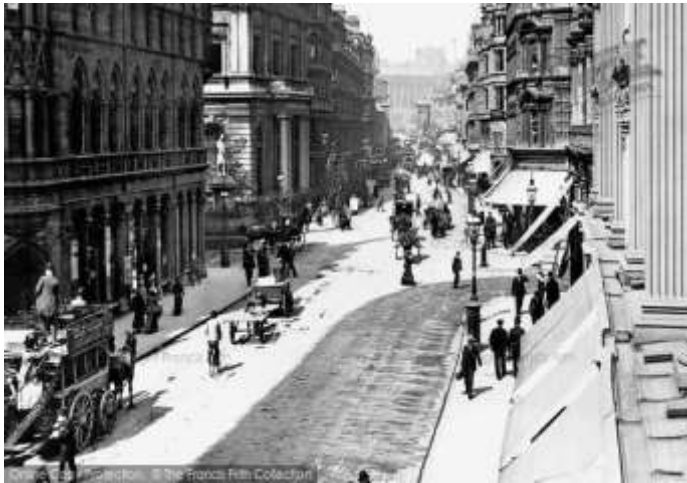
110 New Street was just past the junction with Corporation Street opposite Cannon Street
