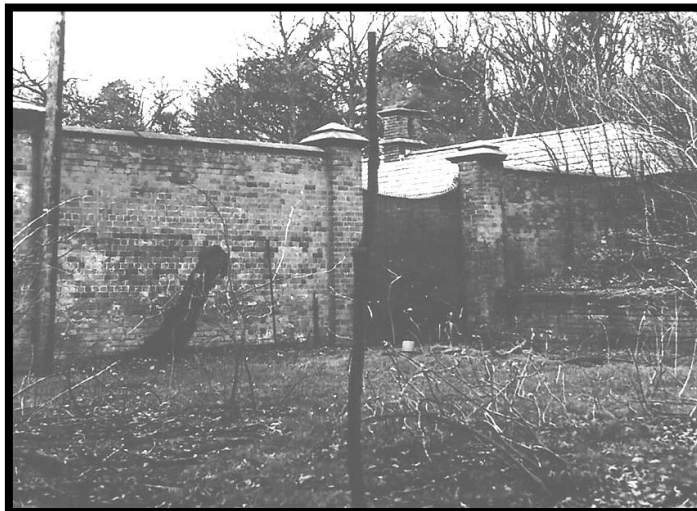
ENTRANCE GATES AND BRICK BOUNDARY WALL TO STABLE BLOCK.
