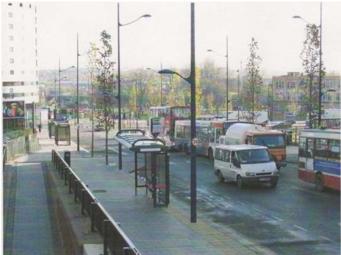
31. View from Priory Queensway, looking towards Moor Street Queensway where Masshouse Circus used to be.
