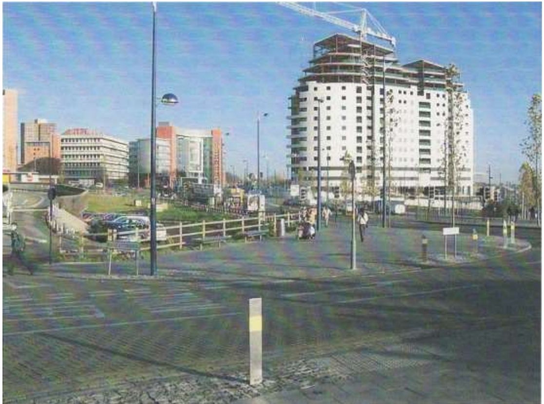
32. Looking towards the junction with Priory Queensway from Moor Street Queensway. Matthew Boulton College can be seen in the centre background and on the right is the first of the new buildings which will eventually transform the new Masshouse area.
