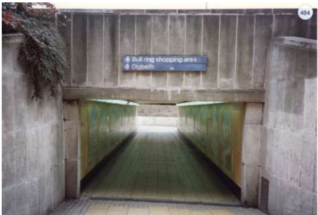
68. Subway beneath Moor Street' Queensway, leading to Moor Street Station.
