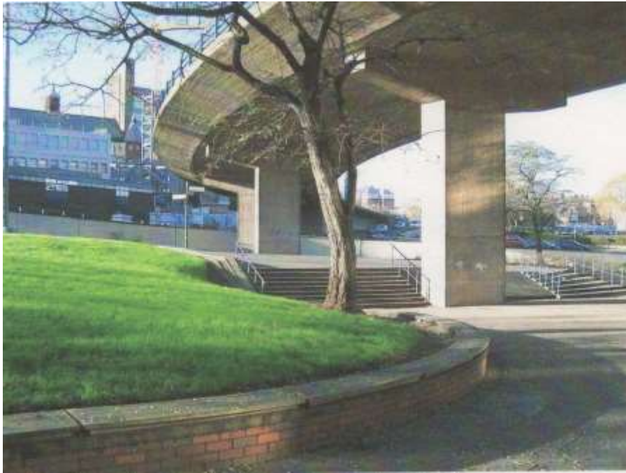
29. Lancaster Circus, showing elevated section of the Aston Expressway.
