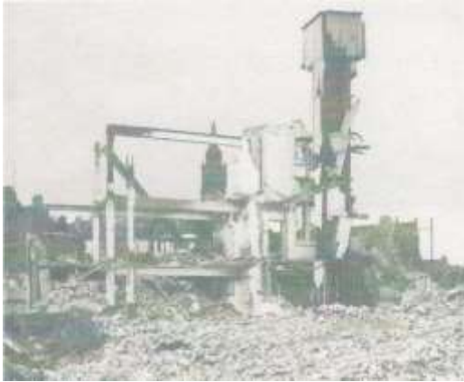
2. Demolition in Progress circa 1963.
