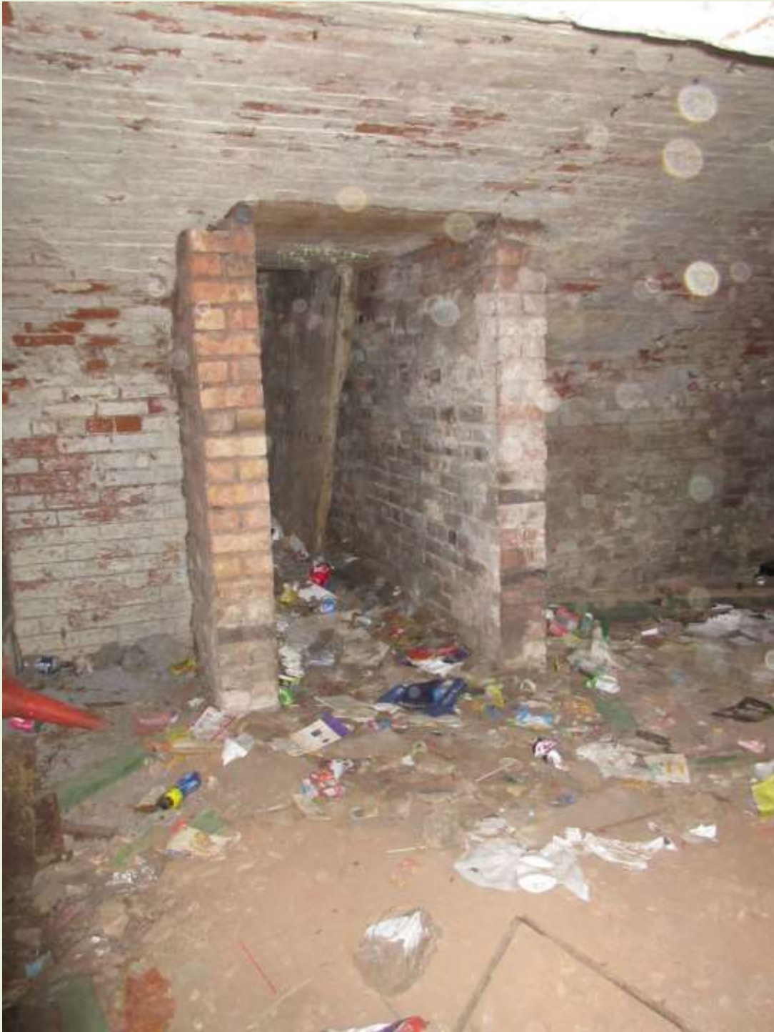
Entrance into the lobby seen from inside the caverns, showing ramp propped up against the wall at the foot of the stairs. The facing wall seems to be the Churchyard boundary. The rubbish appears to be recent (probably accumulated after the green door was removed). (JJ)
