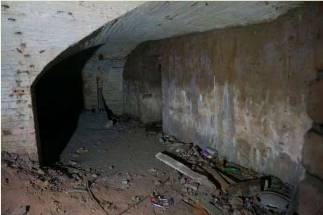
Straight ahead view from lobby entrance into the caverns. Coleshill Street to the right. The plastered wall seems to follow the Vesey Memorial Garden wall above it, fronting Coleshill Street. At the top left of the photo is a row of reinforcing rods in the ceiling of the first cavern, first room, which leads off from the left of the photo. (ED)
