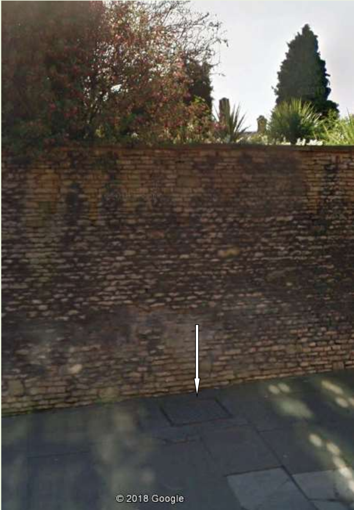
Pavement in Coleshill Street showing manhole cover above chamber. (Google Earth)
