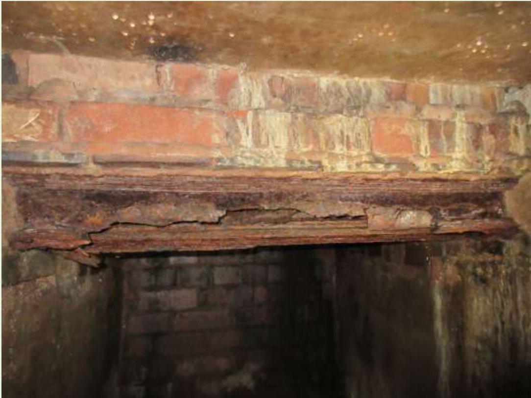
Corroded lintel supporting chamber wall. (JJ)
