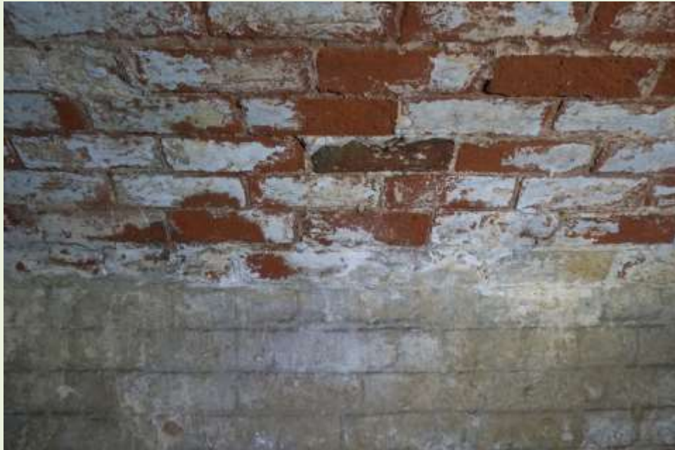
Junction of wall and vaulted ceiling, showing two sizes of brick. The grey wall bricks are thinner, leading one to think the vaulted ceiling was built much later (perhaps when the Vesey Memorial Gardens were built). (ED)
