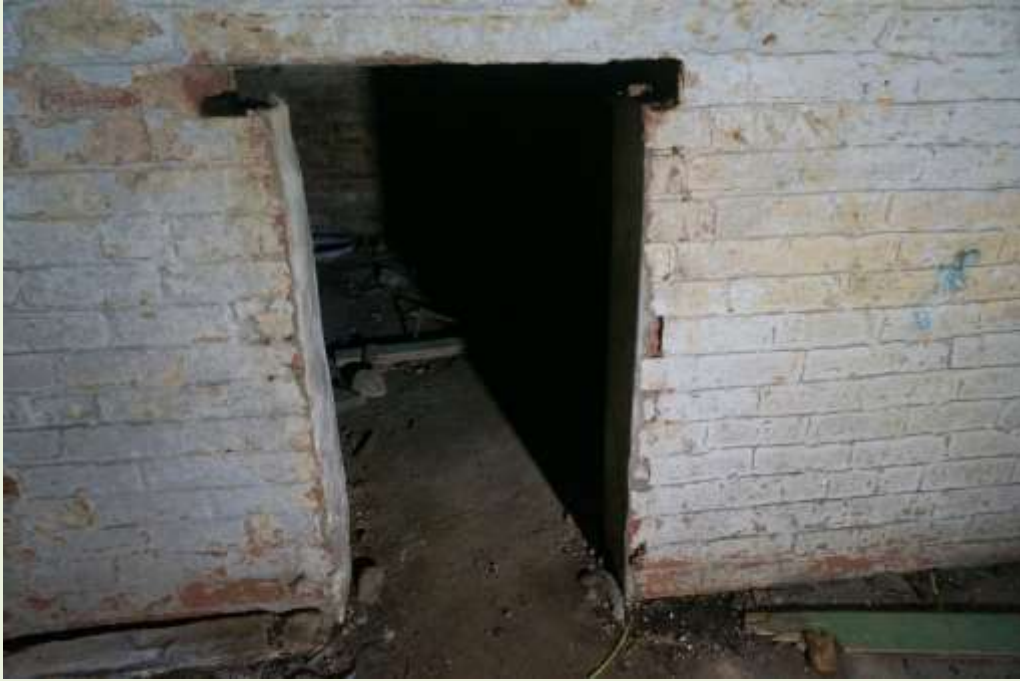
Interconnecting doorway between rear rooms of first and second caverns. Wooden lintel is possibly on the floor (ED)
