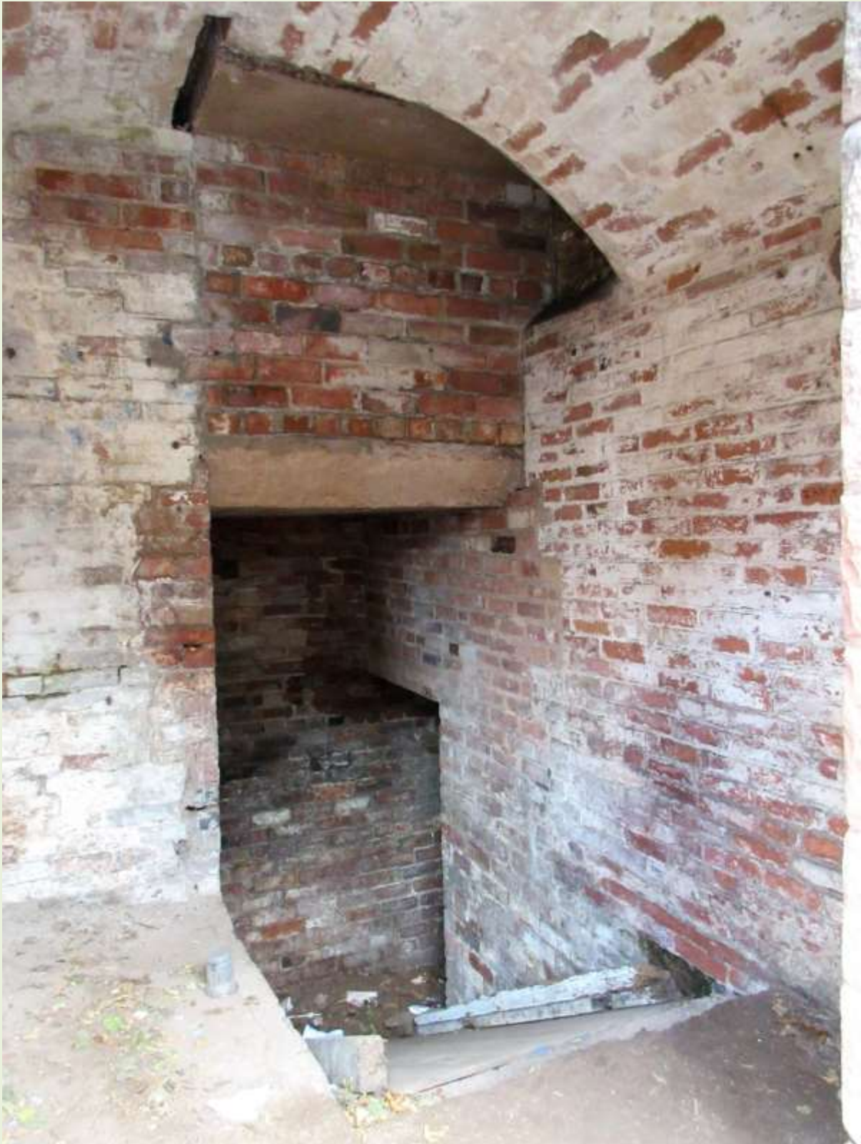
A closer view of wooden ramp leading downwards and the overhead access way into the lobby. (JJ)
