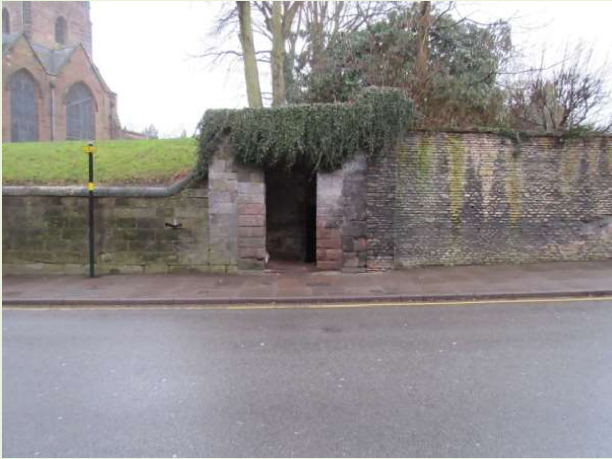
Lobby dooway, showing a variety of brick surrounds and the grassed area above the roof, 2018 (JJ)
