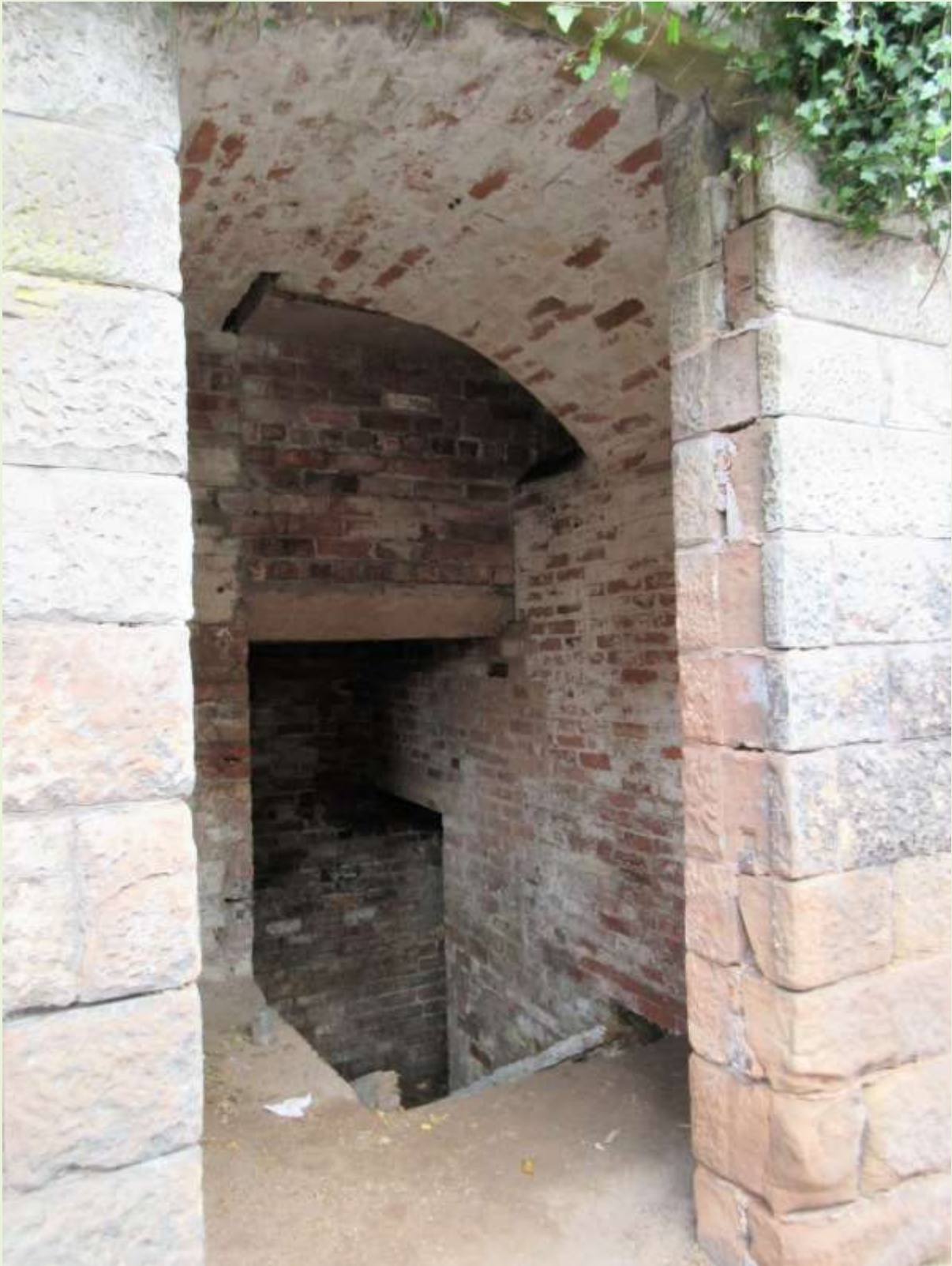
Photo taken of the lobby entrance, showing the overhead access way, the wooden ramp over the stairs leading downwards and the underground doorway leading to the right into the caverns. (JJ)
