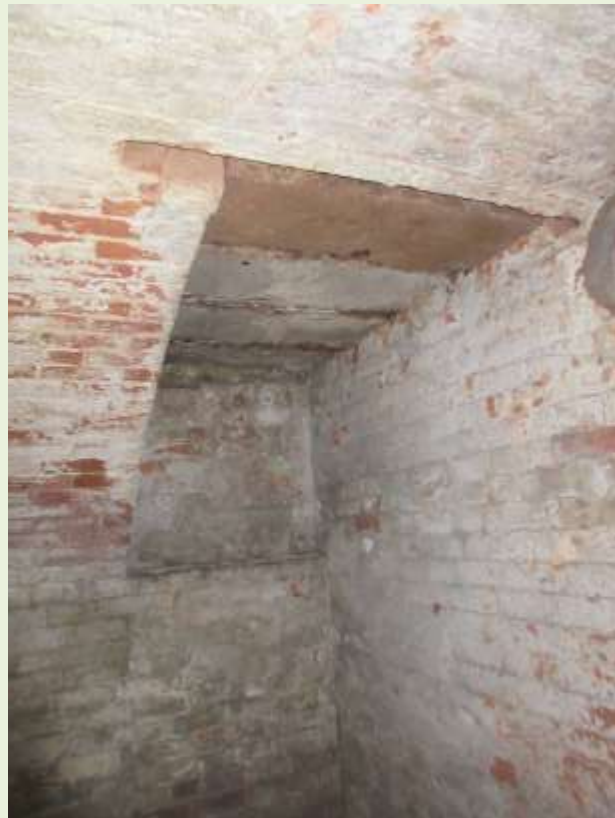
First cavern, rear room, entrance from the roof, probably a stairwell, showing whitewashed ceiling (for light). (JJ)
