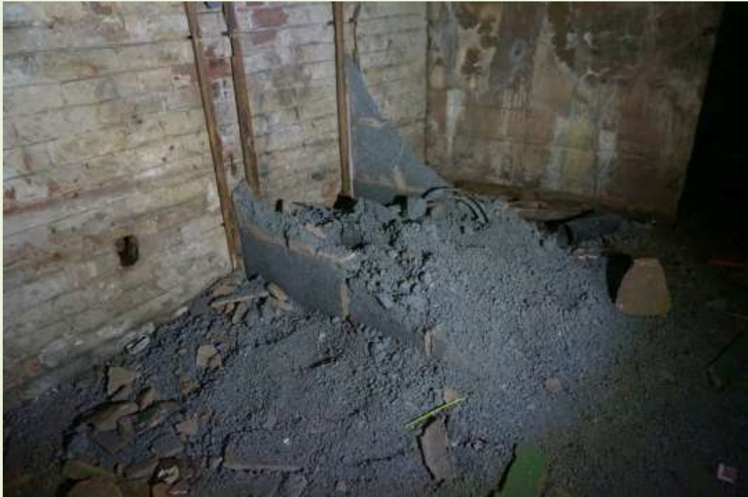
Second cavern. A pile of ash, or broken breeze blocks?(ED)
