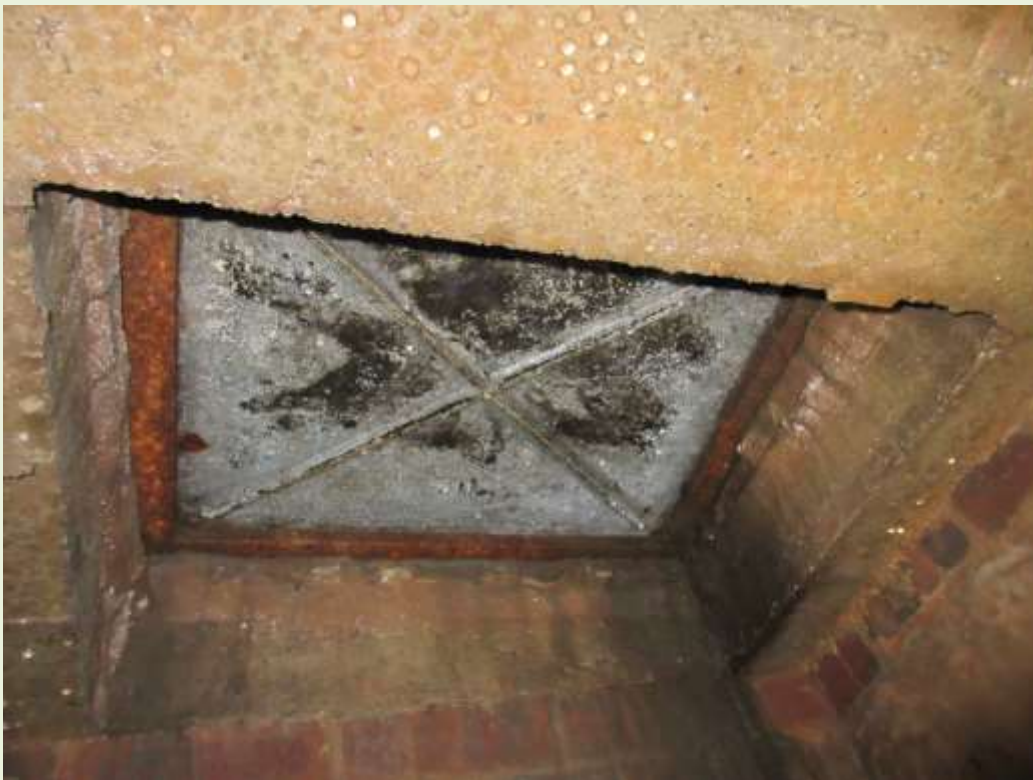
The metal manhole cover in the pavement, seen from below. (JJ)
