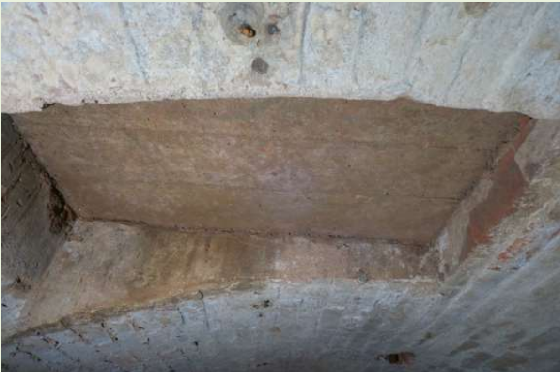
Blocked up entry in roof of first cavern, first room, the stairwell leading downwards from the former dwellinghouse above. (ED)
