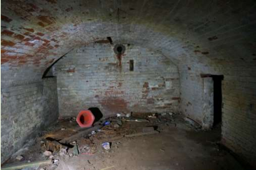
First cavern, rear room, showing a rather short interconnecting doorway to a second cavern, a former entrance into the cavern from the roof on the left hand side and the stairwell from the former dwellinghouse above. (ED)
