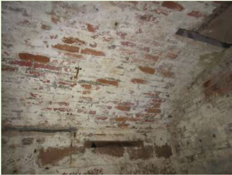
Vaulted roof of lobby, with the boarded up overhead entrance. This structure sits under the grassed over churchyard. The lobby entrance is to the left of the photo. (JJ)
