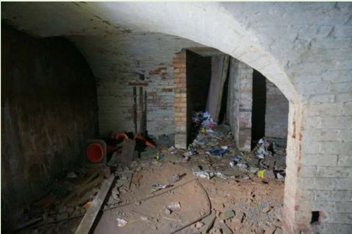
View from second cavern looking towards the lobby with ramp propped up at the foot of the stairs leading to the street above (ED)
