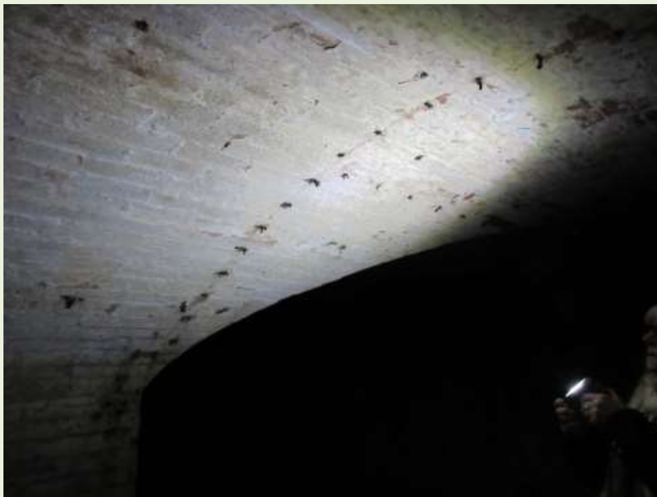
Metal reinforcing rods inserted in roof of first cavern, first room. (JJ)
