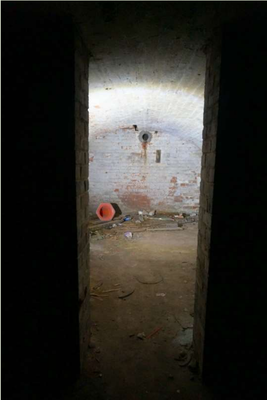
First cavern, looking into rear room with old pipe in rear wall. (ED)
