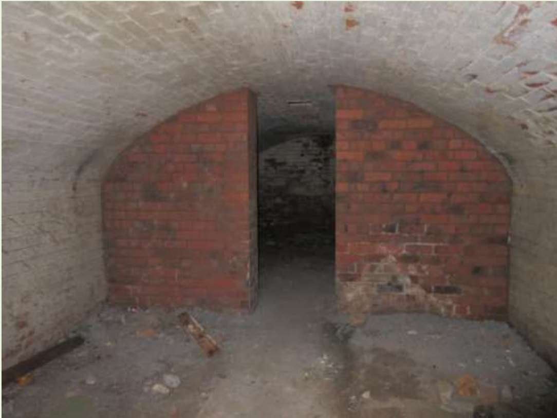
Second cavern, looking towards the rear room with dividing wall (perhaps a strengthening wall inserted at the time Vesey Memorial Gardens were made?) (JJ)
