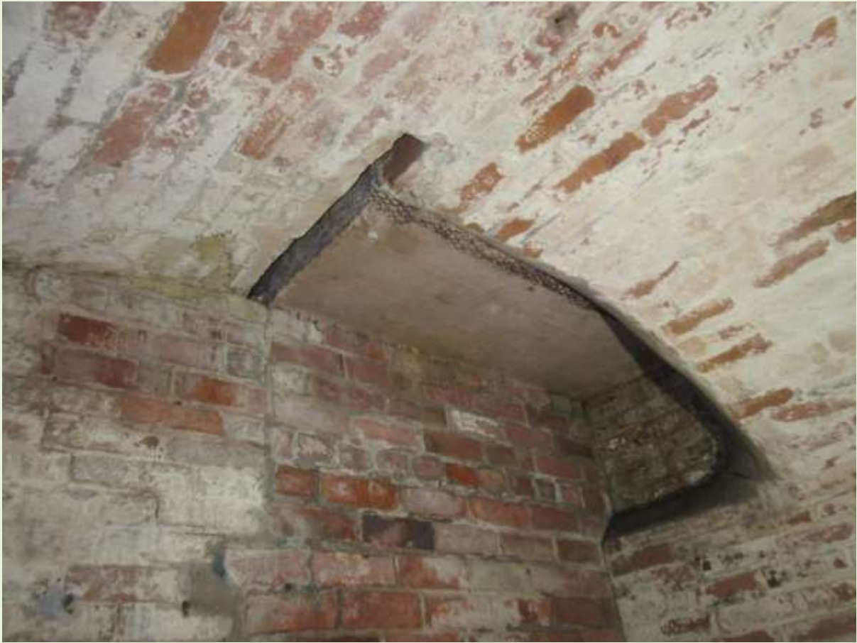
Roof of Lobby, showing a boarded up overhead entrance, possibly a former access from the dwellinghouse above. (JJ)
