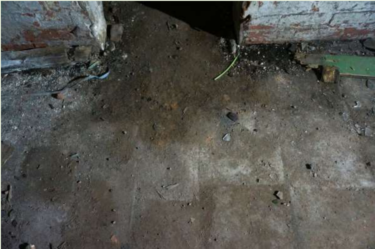
Large tiles on the floor in front of the interconnecting doorway. (ED)
