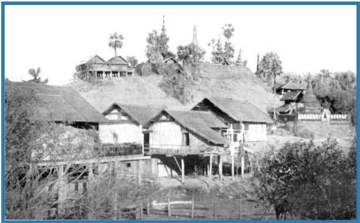
10. Burmese Houses built on piles
